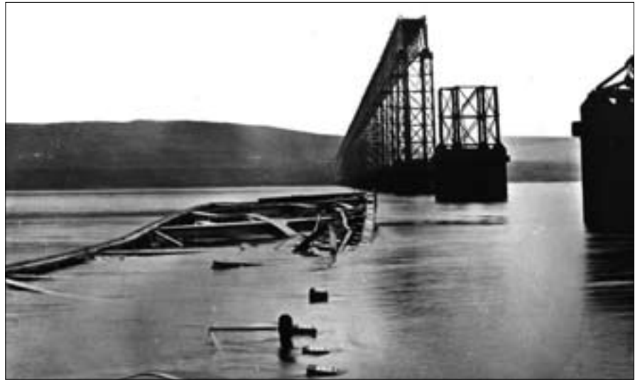
Tay Bridge, at Dundee, Scotland, was also ultimately a victim of metal fatigue in cast iron, according to Peter Lewis. It collapsed in 1879, claiming 75 lives. (Photograph courtesy of Peter Lewis.)
