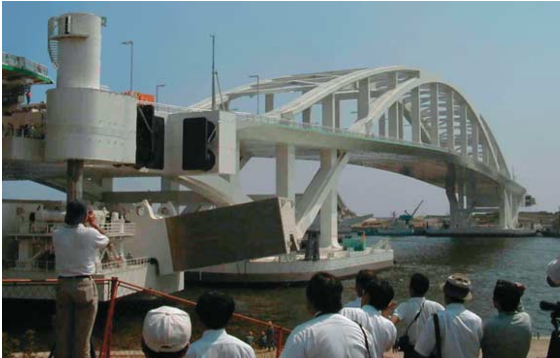
Figure 4. Osaka Harbor's Yumemai Floating Bridge is the world's first swinging floating bridge. (Images in Figures 4 and 5 courtesy of Eiichi Watanabe, Kyoto University.)
