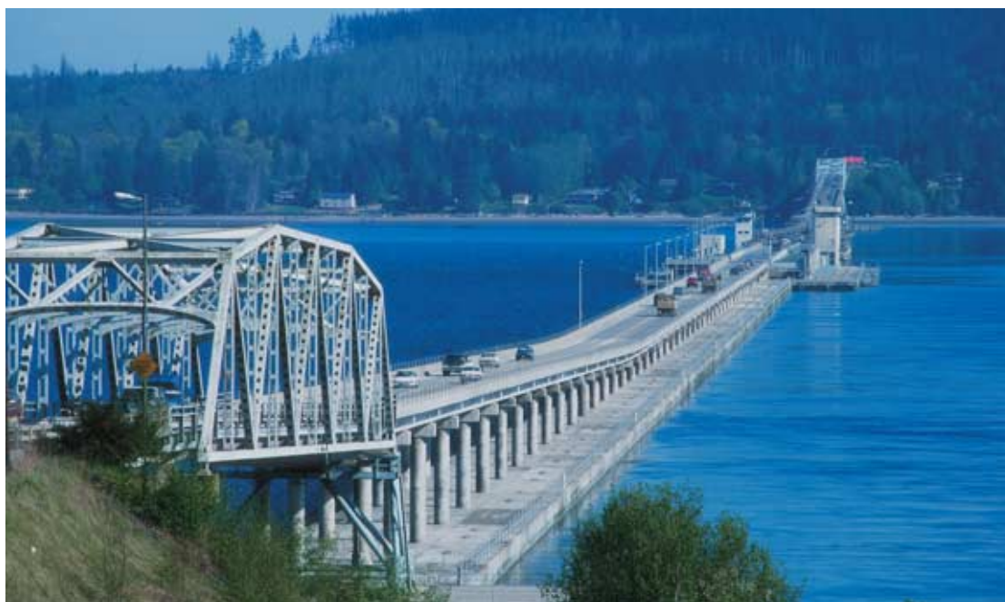
Figure 3. Hood Canal Floating Bridge incorporates a unique "sliding" section to allow vessels to pass.
