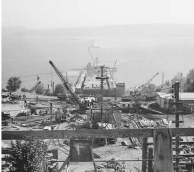
Figure 2. Originally known as the Mercer Island Bridge, the Lacey V. Murrow Bridge was built using concrete pontoons.
