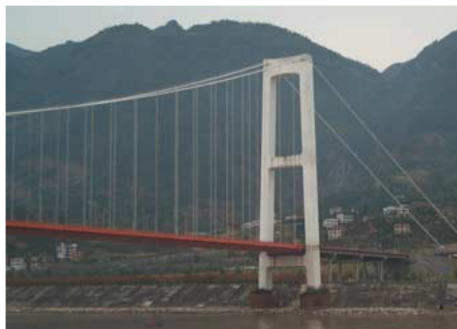
Figure 4. Xiling Bridge crosses the Yangtze just downstream from the Three Gorges Dam site. (Photograph courtesy of Catherine Petroski.)
