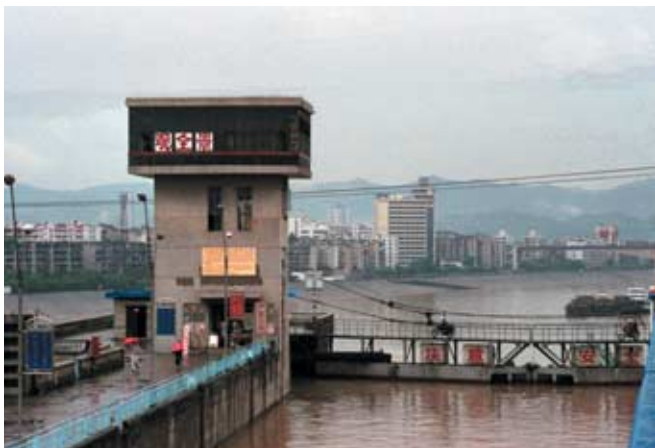
Figure 3. Lock at Gezhouba Dam, completed in 1981, provides shipping access above Yichang. (Photograph courtesy of Alan R. Miller.)
