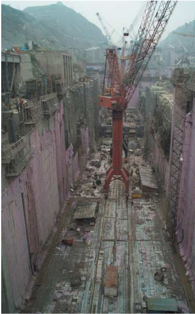
Figure 4. Ship locks for Three Gorges Dam have been carved out of solid granite. (Photograph courtesy of Catherine Petroski.)
