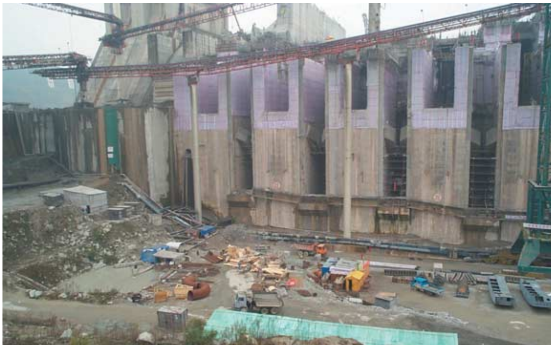
Figure 6. Large trucks are dwarfed by the rising concrete gravity dam. (Photograph courtesy of Catherine Petroski.)
