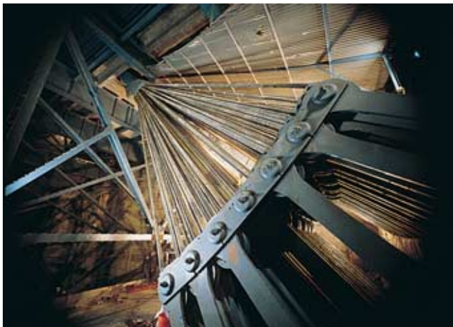
Figure 3. Cables were spun in place, and each consisted of more than 20,000 individual steel wires—twice as many as any previous bridge. (Photograph courtesy of James B. Abbott.)
